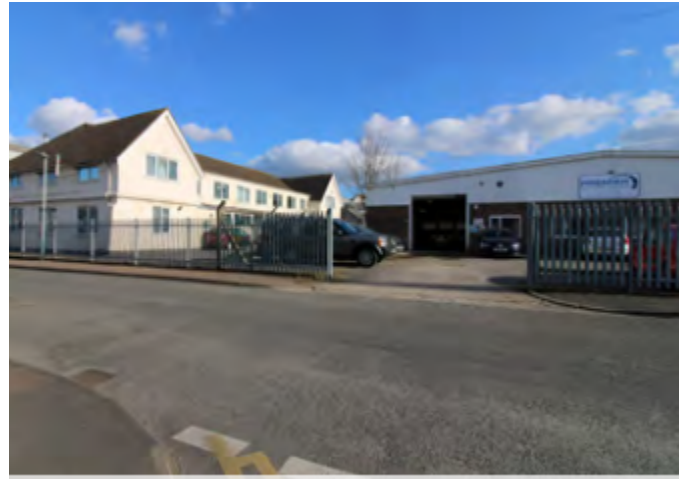
8: View towards industrial unit access road at western site boundary
